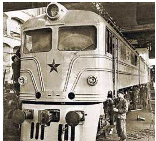
NV 001 electric locomotive in the NEVZ' assembly shop
